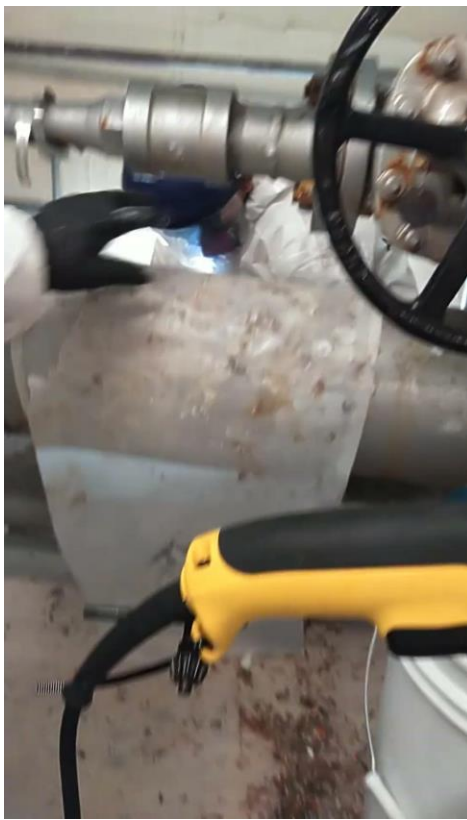
HAZMAT lead pipe paint removal-SRP Canyon Lake facility
